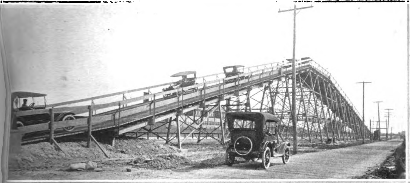
Dodge Bros., Detroit, Mich., have completed a 1/2-mile speedway, test hill and sand pit on the factory grounds for the purpose of keeping their test men off the public streets and roads. The hill is 542 ft. long by 30 ft. wide and has two approaches with varying grades. Over 215,000 ft. of lumber is used in the track, on which no pedestrians are allowed
